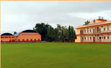
INDOOR KHO-KHO & DRESSING ROOM
